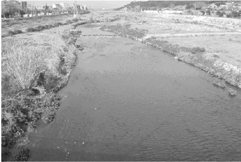
Figure 2: Besòs river in the area of study. Canalized river channel, scarcity of meanders and concrete walls delimiting the flooding zone may be seen.
